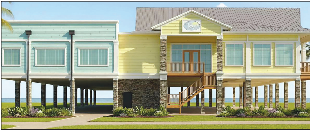
Roy's released a rendering of its architect's conceptual design (above) of the new restaurant online in February, showing the new facility will be constructed on pilings some 19 feet above mean sea level (approximately 15 feet above the ground) – with stairs and an elevator – making it fully handicapped accessible and in compliance with current building codes.
